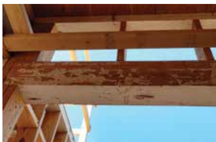
Surfaces can erode, chip, flake, and break down over time. Be sure to use fire-retardant-treated-wood that meets code requirements for project specifications.
