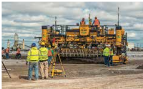
Topcon's Millimeter GPS and LPS system allows a crew to pave 52 lanes of concrete without using a stringline.
