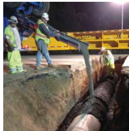
Granite Construction and subcontractors using the MBT-1 in California (above) and Washington (below). Caltrans called for barrier in its specifications and the MBT-1 proved a most efficient tool. WSDOT provided the barrier for use by the winning bidder as part of a project there.
